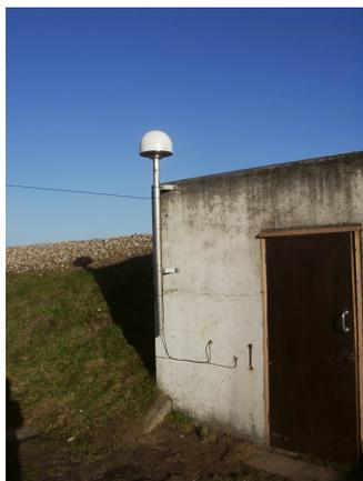
Figure 3. Antenna installation at a remote station.
